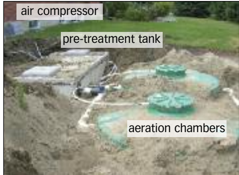
Large sewage design flows may require more than one aeration chamber.
