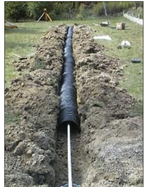
Single line shallow buried trench.
